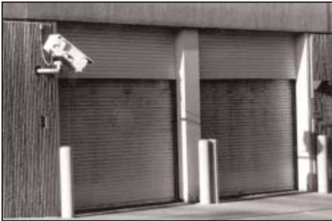
CCTV monitors cars entering and leaving this garage.
