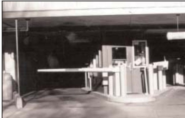
Attendants and electronic barriers provide good control of the exit at this deck.
