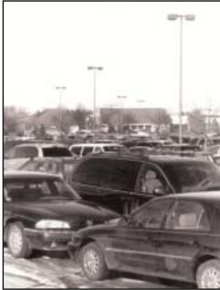
Tall lights provide uniform coverage of a lot and are difficult to vandalize.
